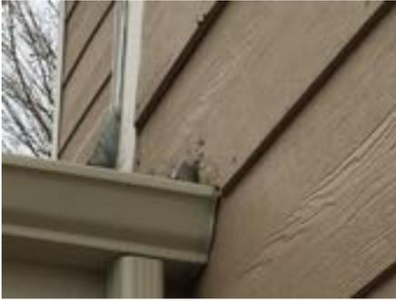
3.01.2 • Wire entry and gas line entry on side of house were not caulked, this may allow moisture penetration and begin delaminating the siding. A qualified contractor should evaluate and repair or replace as necessary and according to current standards.
