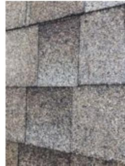
1.07.2 • The subjects roof had signs of shingle cracking and random areas of damage indicative to hail. A qualified contractor should evaluate and repair or replace as necessary and according to current standards.
